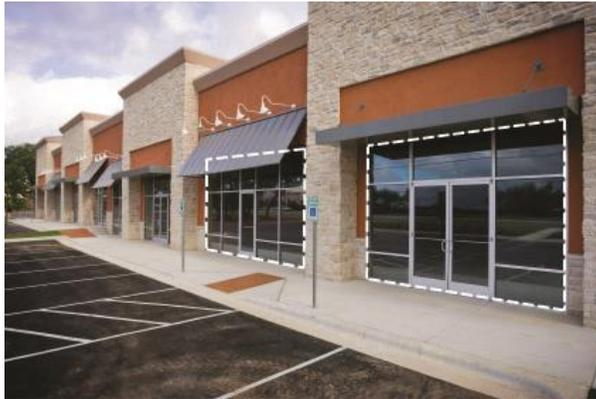
Figure 1123-E: The window area is illustrated within the dashed line area for the two storefronts in the above image.
