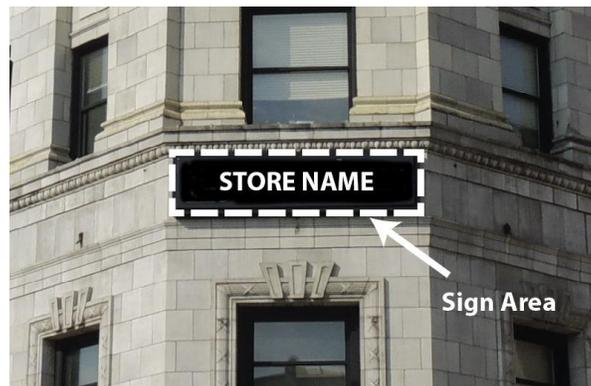
Figure 1123-B: Illustration of computing the sign area for wall signs with a background panel or cabinet.
